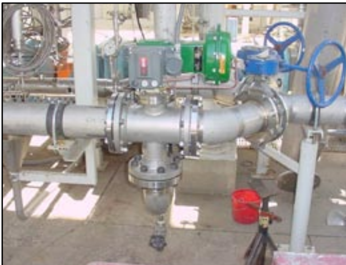
Above: Solaris in a hot break installation.
